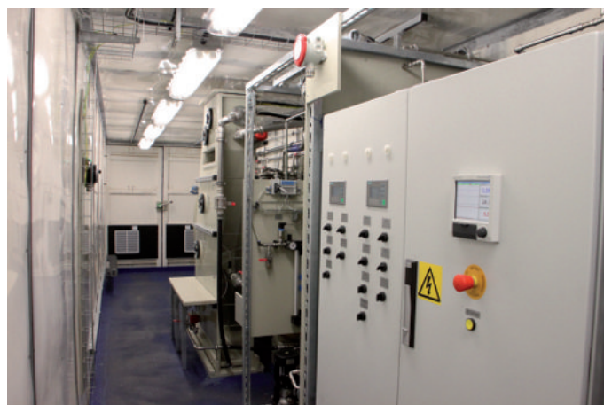
The fully automated OilPaq is controlled by means of a touch screen and is housed in aerated office containers.
